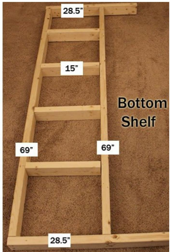
Build the top frame and bottom shelf as outlined and connect the 2x4 pieces using 3 inch #10 construction screws.
